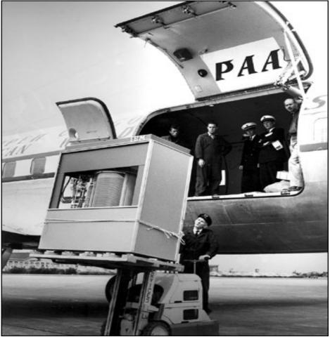
This IBM 305 RAMAC Computer, introduced in 1956, was the first computer containing a (5 MB) hard drive on 24 huge spinning platters. Today you can get 1000 times more memory in something the size of your thumb.
