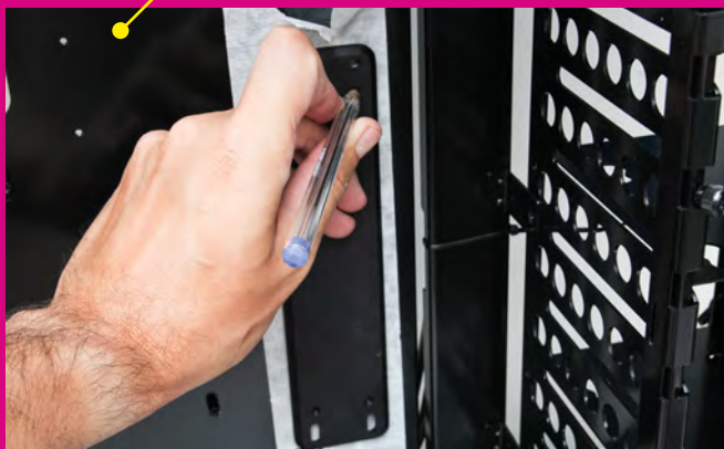
Mark up where you need the holes using masking tape and a pencil
