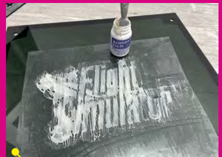
Apply the etching cream using a brush and leave it on the glass for the specified amount of time
