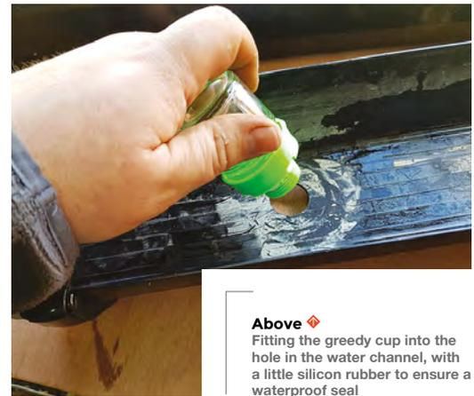
**Above** ◆ Fitting the greedy cup into the hole in the water channel, with a little silicon rubber to ensure a waterproof seal
